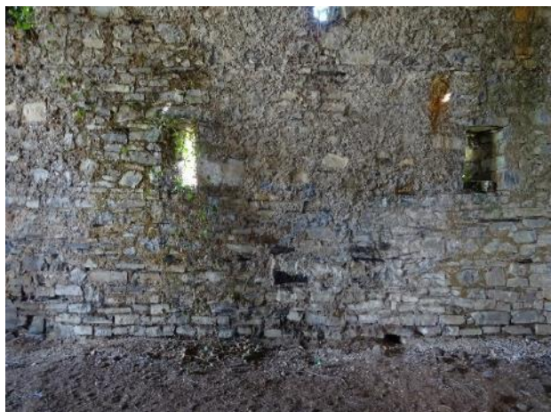
Fig.64: Coach House, west section, north internal elevation, missing stone at the bottom section and stains from the corrugated metal sheeting.
