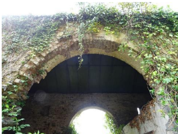
Fig.49: Coach House, West section, external north elevation, western opening, missing bricks and stones.
