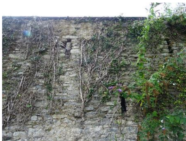
Fig.33: Coach House, west section, north elevation, stone have fallen at the window opening, vegetation overgrowth.
