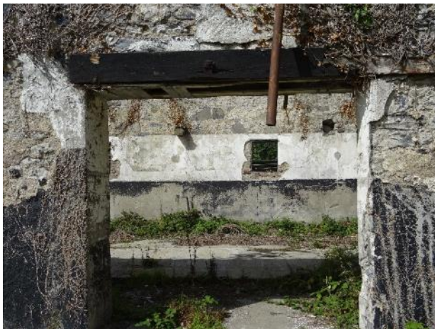
Fig.11: Barn, external south elevation, square-headed door opening with concrete lintel and reveal.
