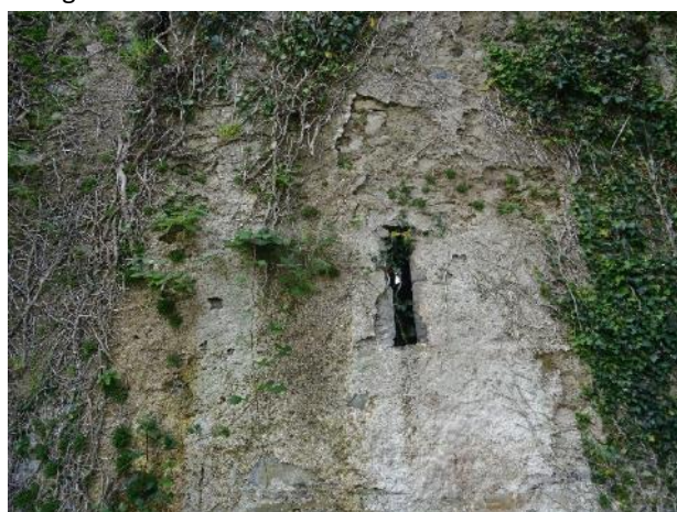
Fig.33: Coach House, west section, north elevation, stone have fallen at the window opening, vegetation overgrowth.
