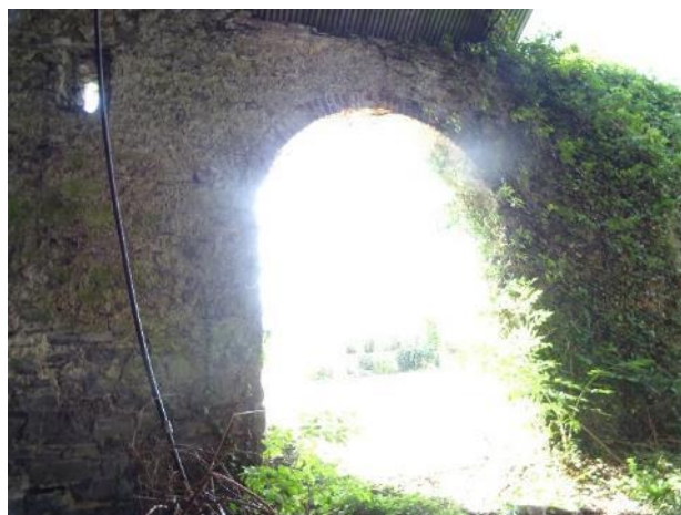
Fig.52: Coach House, West section, internal south elevation, western opening, missing stones at the base of the arch.
