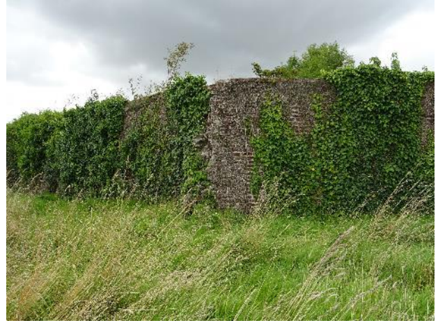
Fig.95: West wall of Walled Garden, brickwork have collapsed.
