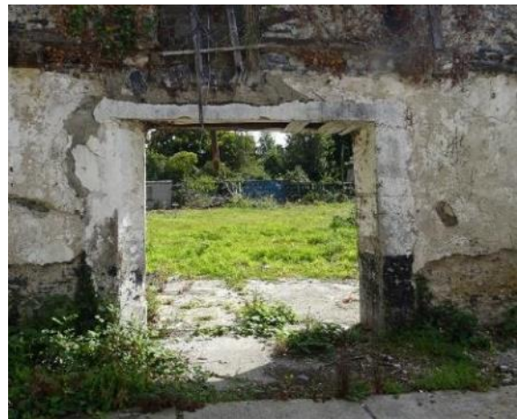
Fig.12: Barn, internal south elevation, square-headed door opening with concrete lintel and reveal.
