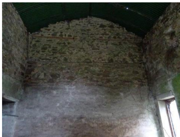
Fig.71: Coach House, west section, west internal elevation, late wall addition
