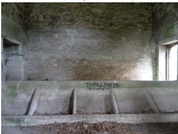
Fig.70: Coach House, west section, south internal elevation, window opening was blocked up.
