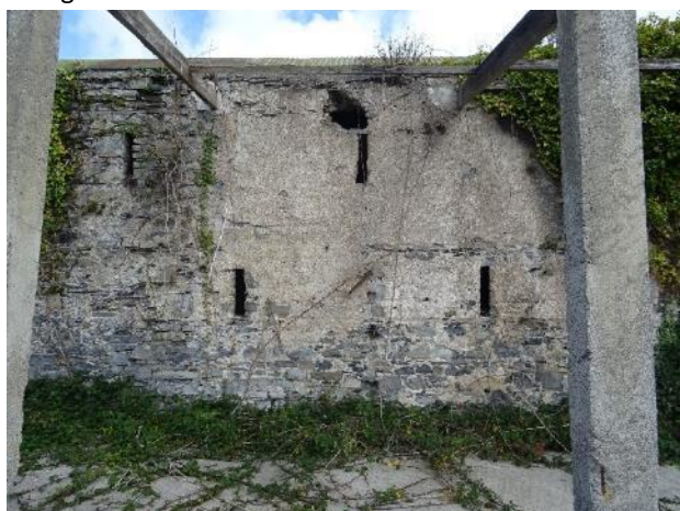
Fig.36: Coach House, west section, south elevation, section at the west has a concrete render, vegetation overgrowth.
