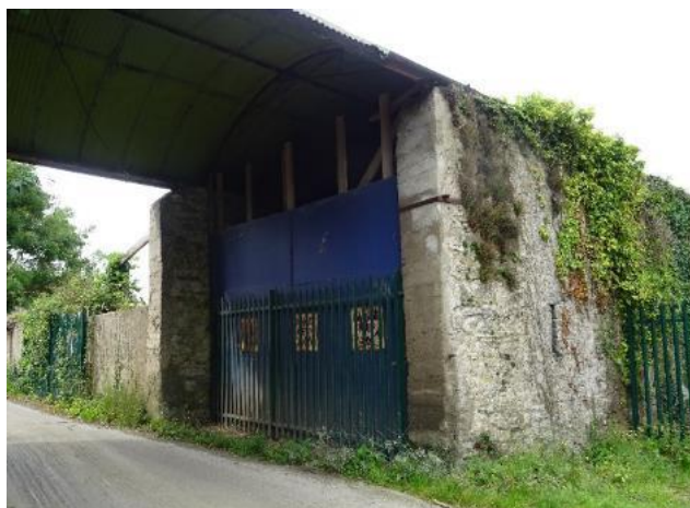
Fig.32: Coach House, west section, north elevation concrete was cast in situ, vegetation overgrowth.
