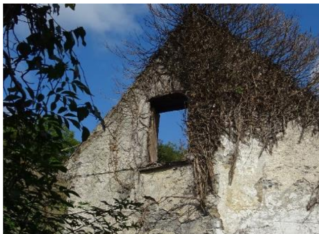
Fig.8: Barn, south elevation, low arch window opening with brick lintel.
