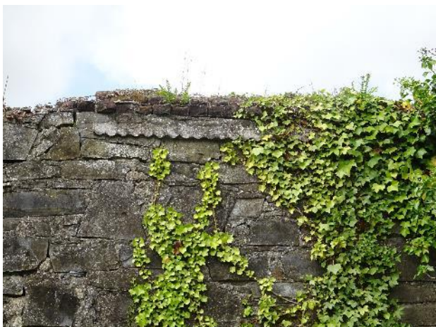
Fig.82: Wall, remaining mortar flashing between roof of the former 19th C building.
