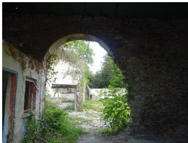
Fig.50: Coach House, West section, internal north elevation, western opening, missing bricks and stones.
