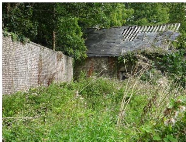
Fig.4: Barn, remaining section of the roof at the north.
