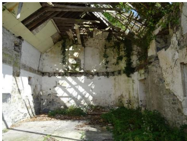
Fig.19: Barn, internal north elevation.
