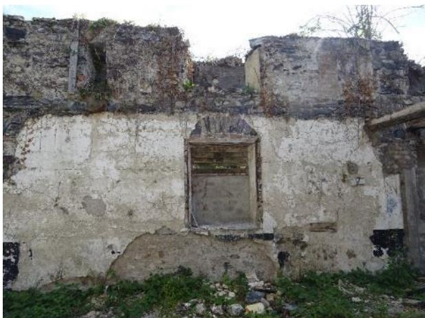
Fig.16: Barn, internal west elevation, concrete render and bitumen paint, timber beam section inserted in the wall indicate that there was previously a floor over the whole layout.
