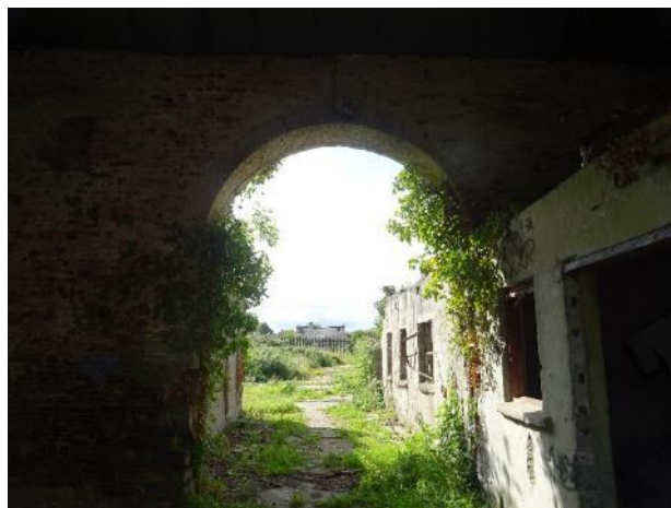
Fig.50: Coach House, West section, internal north elevation, western opening, missing bricks and stones.
