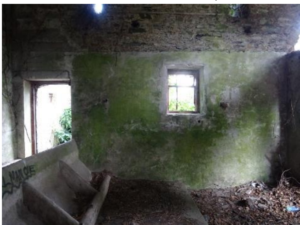
Fig.72: Coach House, west section, west internal elevation, cement render at the bottom part.
