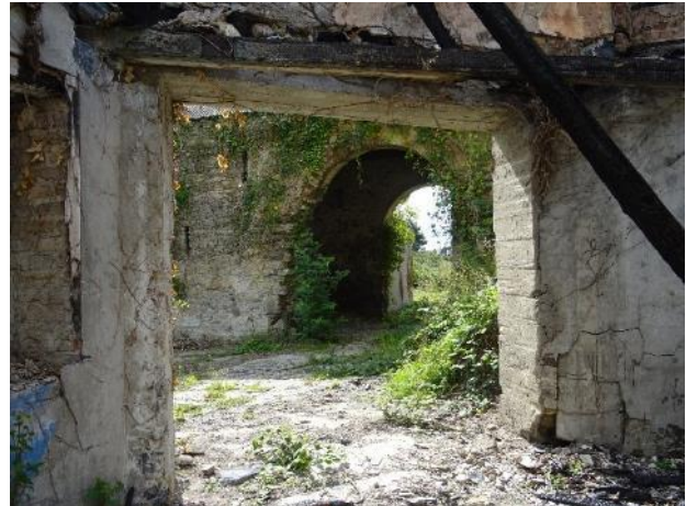
Fig.12: Barn, internal south elevation, square-headed door opening with concrete lintel and reveal.
