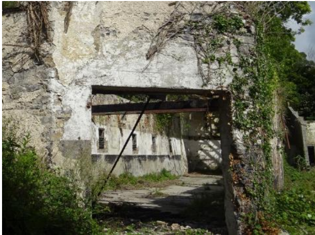
Fig.11: Barn, external south elevation, square-headed door opening with concrete lintel and reveal.
