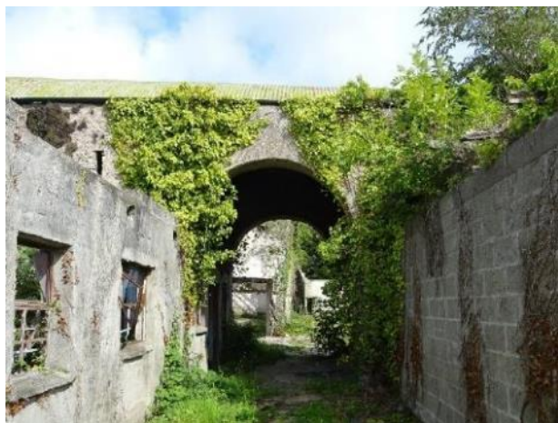
Fig.49: Coach House, West section, external north elevation, western opening, missing bricks and stones.
