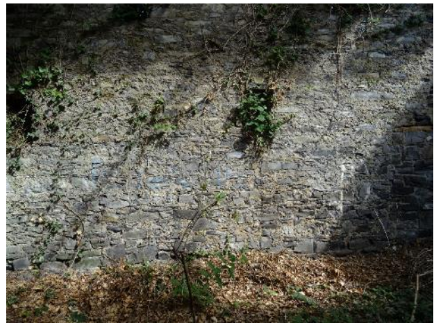
Fig.61: Coach House, west section, north internal elevation, vegetation overgrowth, open joints at the bottom section, graffiti.
