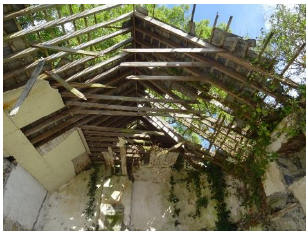
Fig.3: Barn, remaining section of the roof at the north.
