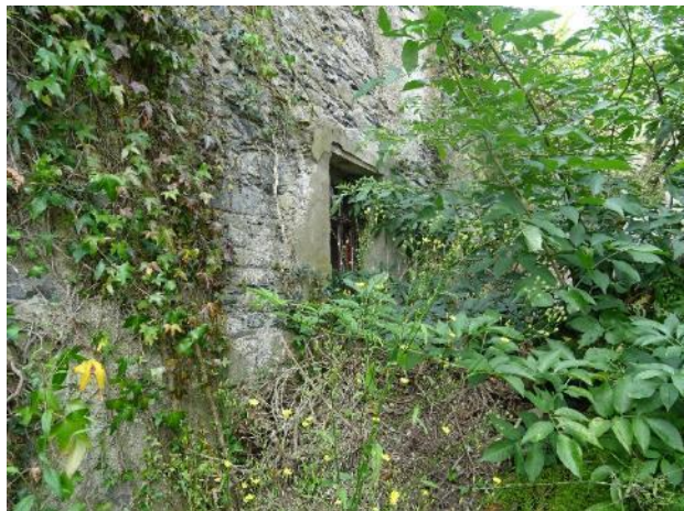
Fig.44: Coach House, west section, external north elevation, non-historic square-headed window.
