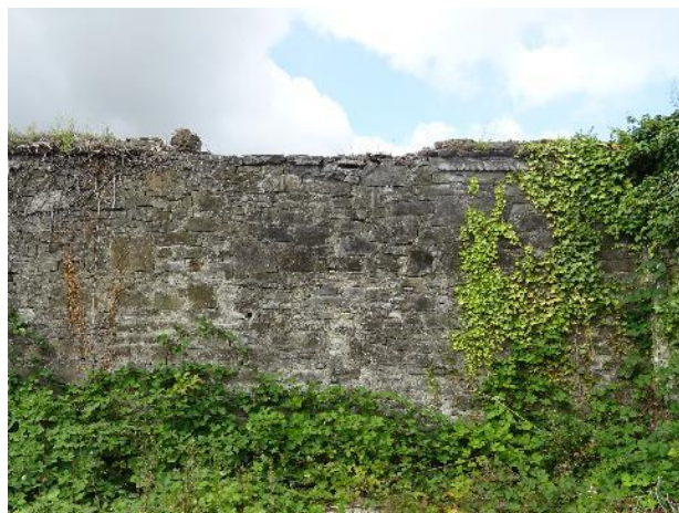
Fig.83: Stone is destabilised where the brickcourse is missing.
