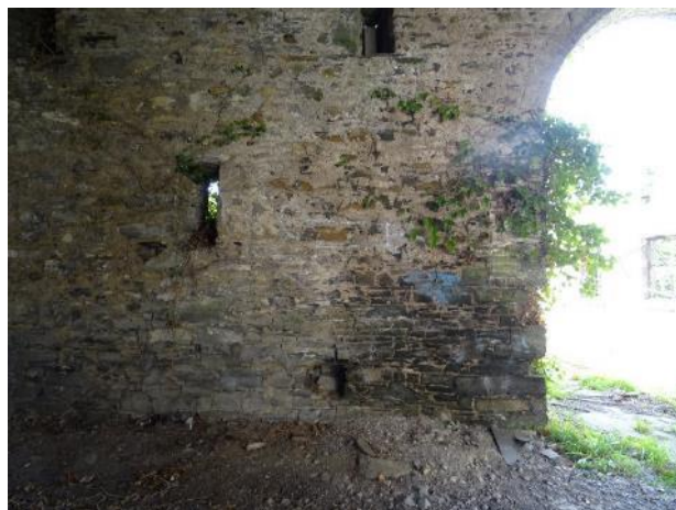
Fig.65: Coach House, west section, south internal elevation, missing stone at the bottom section and crack.
