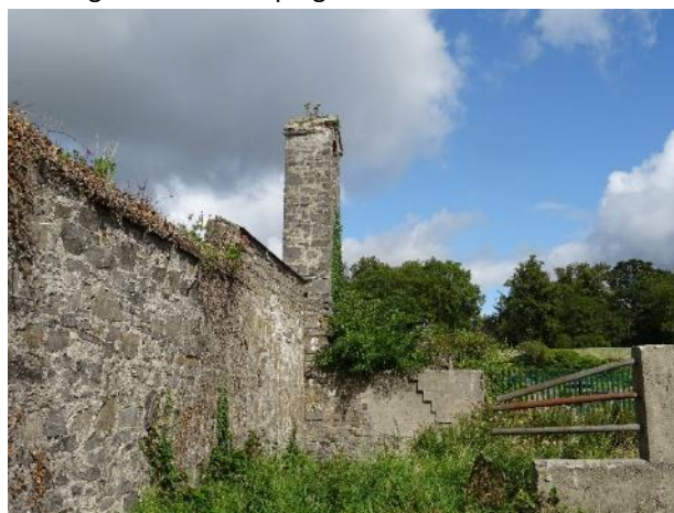
Fig.79: Bell tower, north elevation, missing flaunching and vegetation developing.
