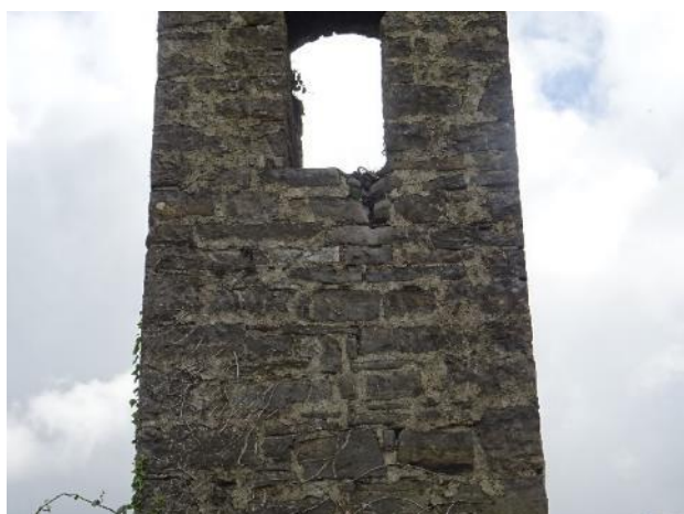
Fig.78: Bell tower, west elevation, missing stone underneath the opening
