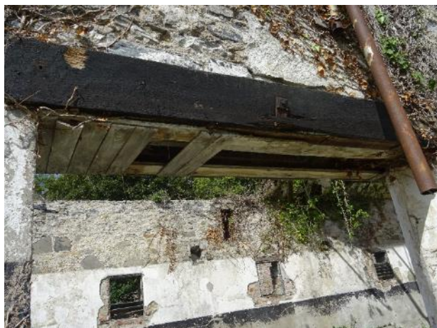
Fig.15: Barn, external east elevation, square-headed door opening with timber beam lintel.
