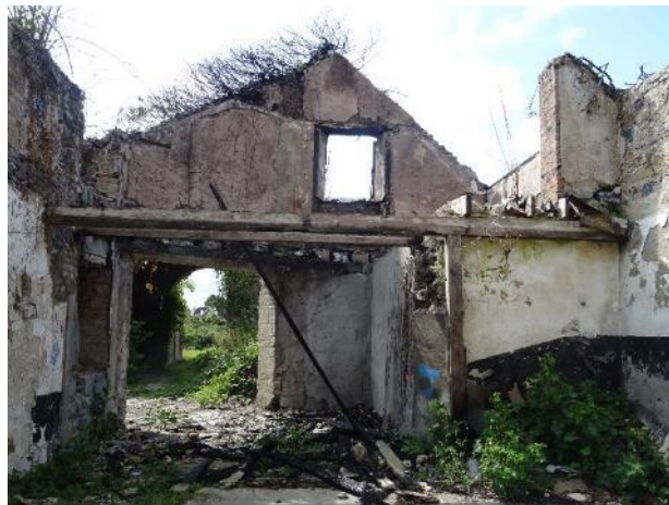
Fig.17: Barn, internal south elevation.
