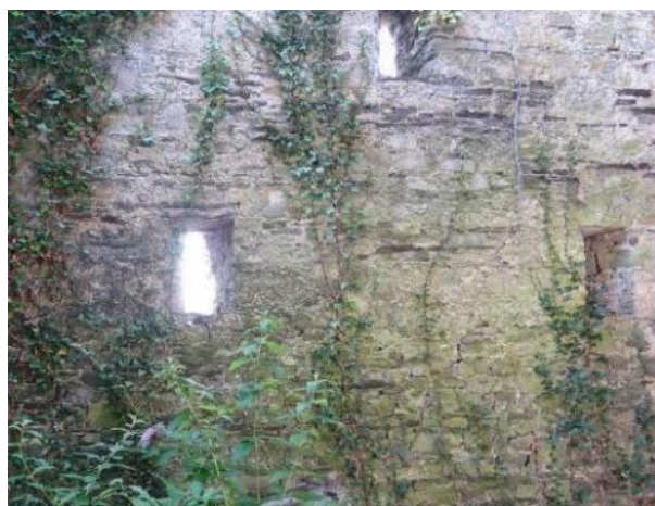
Fig.65: Coach House, west section, south internal elevation, missing stone at the bottom section and crack.
