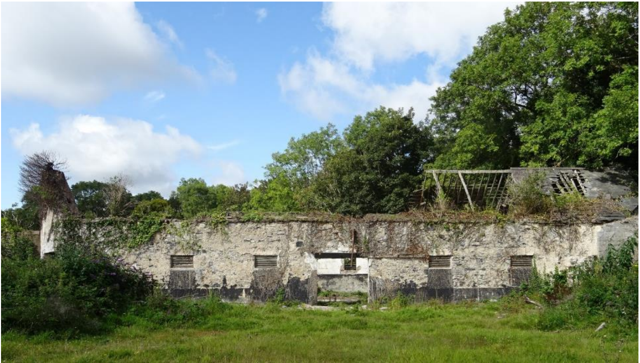
Fig.1: Barn east elevation
