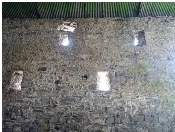
Fig.67: Coach House, west section, south internal elevation, section close to central opening, diagonal crack.
