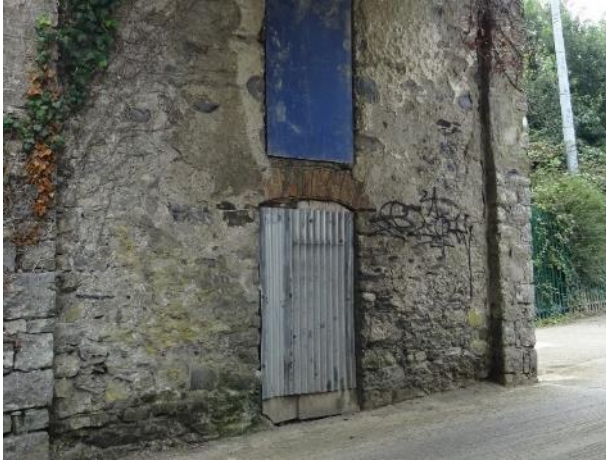
Fig.55: Coach House, east section, west elevation, low arch door opening was boarded up.
