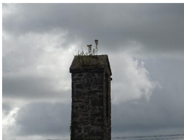
Fig.79: Bell tower, north elevation, missing flaunching and vegetation developing.
