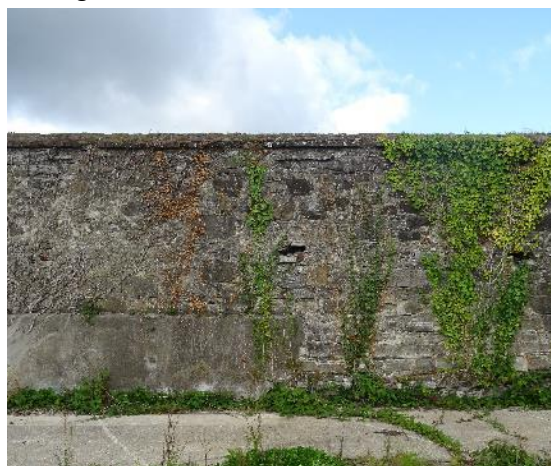
Fig.83: Stone is destabilised where the brickcourse is missing.
