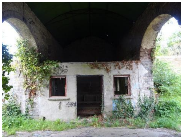
Fig.71: Coach House, west section, west internal elevation, late wall addition
