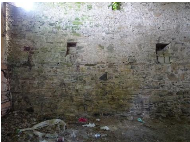
Fig.70: Coach House, west section, south internal elevation, window opening was blocked up.
