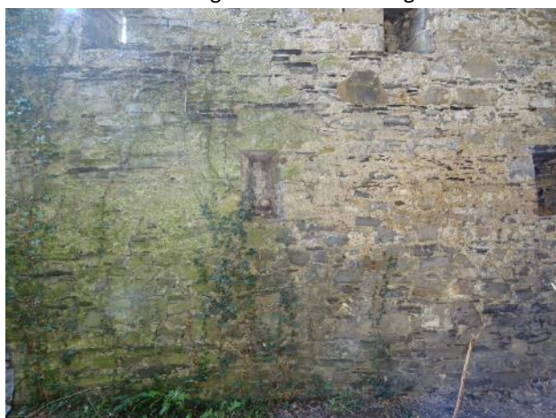
Fig.64: Coach House, west section, north internal elevation, missing stone at the bottom section and stains from the corrugated metal sheeting.
