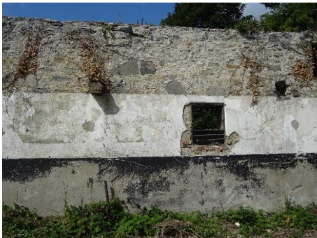
Fig.16: Barn, internal west elevation, concrete render and bitumen paint, timber beam section inserted in the wall indicate that there was previously a floor over the whole layout.
