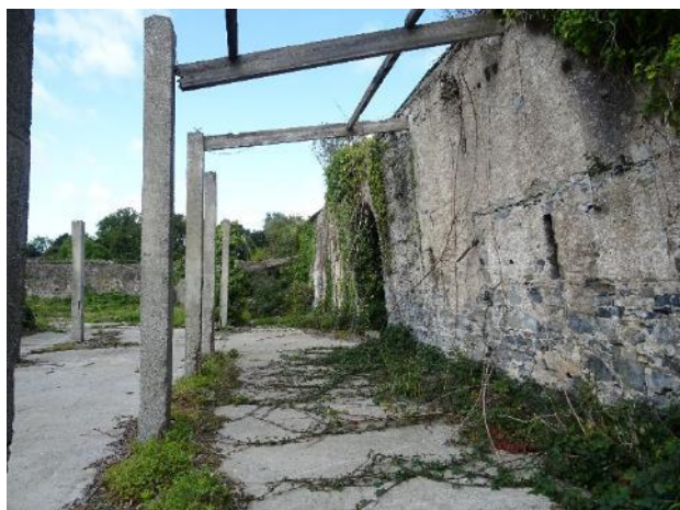
Fig.38: Coach House, west section, south elevation, missing stones, open joints on the top and bottom section, alterations due to the timber beams, vegetation overgrowth.
