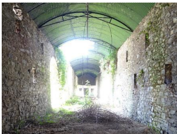
Fig.23: Corrugated steel sheeting supported by curved steel trusses. The roofing is missing at the centre.
