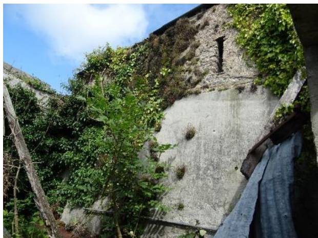
Fig.36: Coach House, west section, south elevation, section at the west has a concrete render, vegetation overgrowth.
